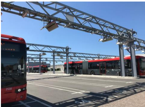
► Pantograph-based charging on racks a) openair-rack infrastructure at Harlem depot (Transdev NL); b) indoor-rack on ceiling, at Eindhoven depot (Hermes/Transdev). Source: A. Abdulah, UITP
