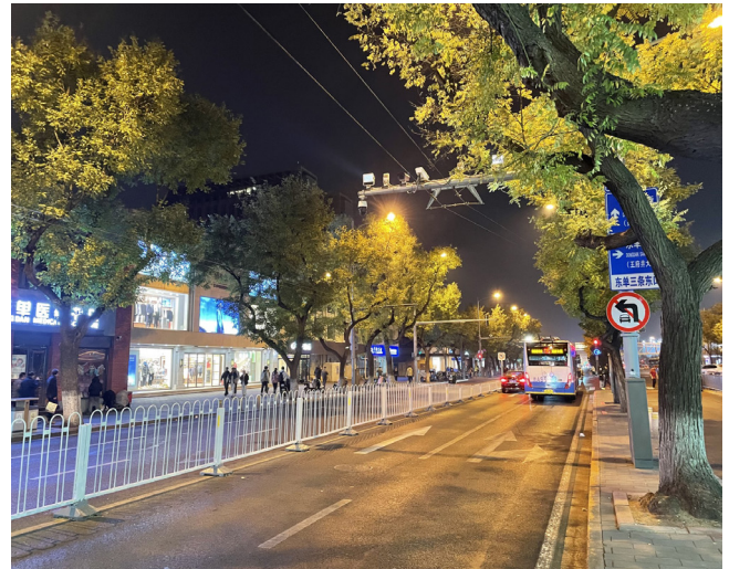
► End of an OCS section on charging road in Beijing, China: Buses de-wire while running. Note OCS visually absorbed by urban tree canopies.
