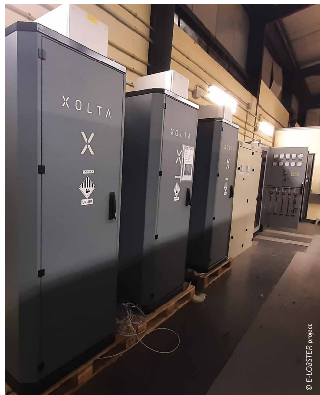
Figure 4: Lithium Balance (XOLTA) modular battery system
