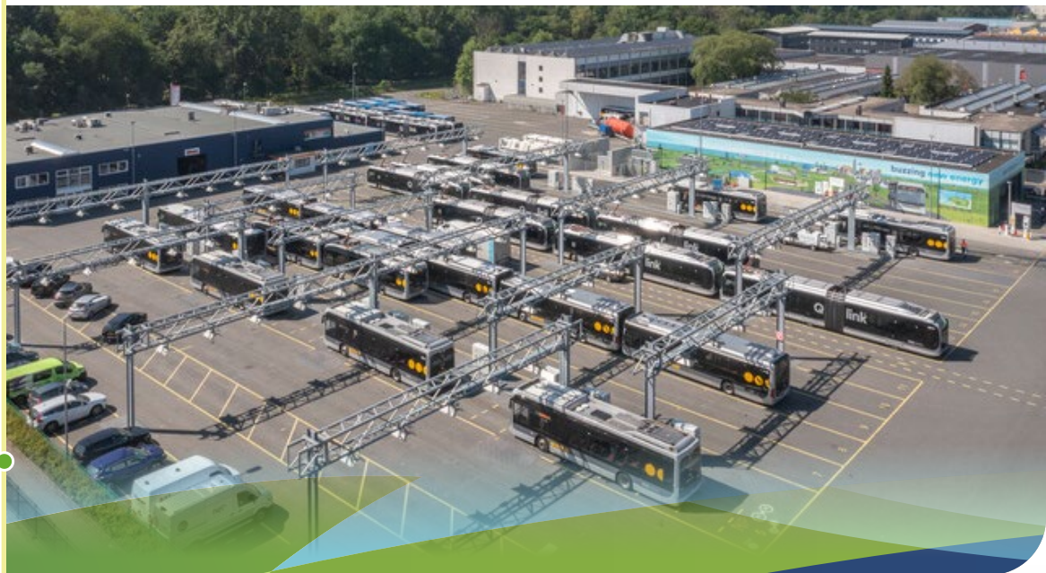
● Depot charging infrastructure in Groningen – Drenthe (Source: OV Bureau Groningen Drenthe)
